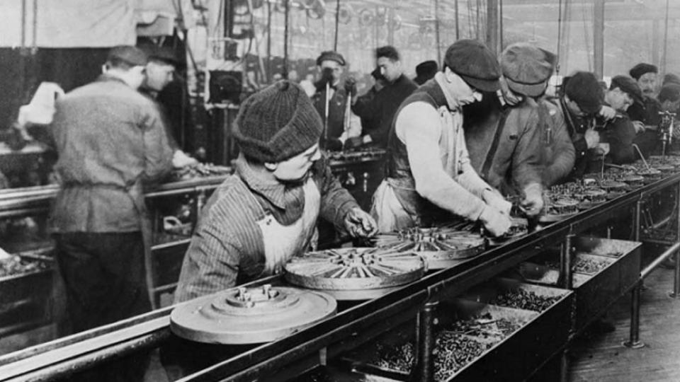
An Assembly Line of the Ford Motor Gompany
